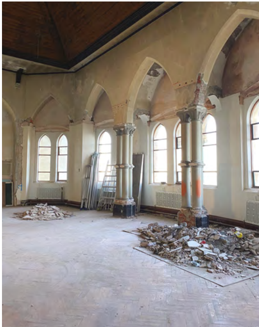
Centre for Dialogue restoration work in progress
