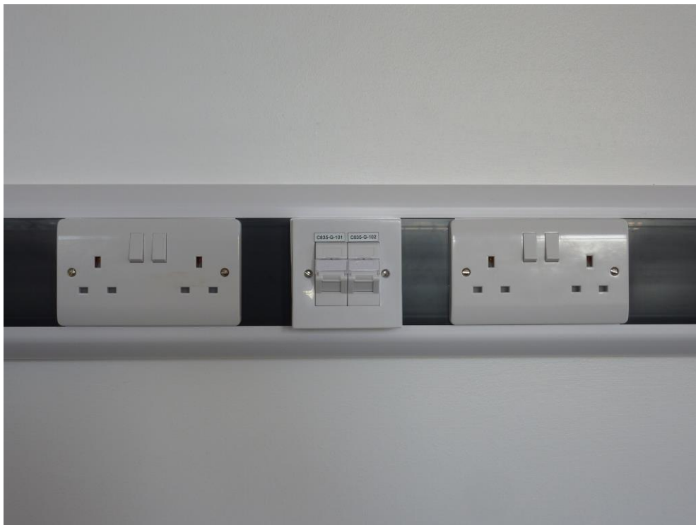
Fig 4.2: Example of the layout of a twin mains, double data, twin mains provision on dado trunking
