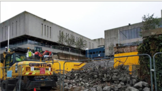
Dismantling the Arts Centre Piazza bridge
